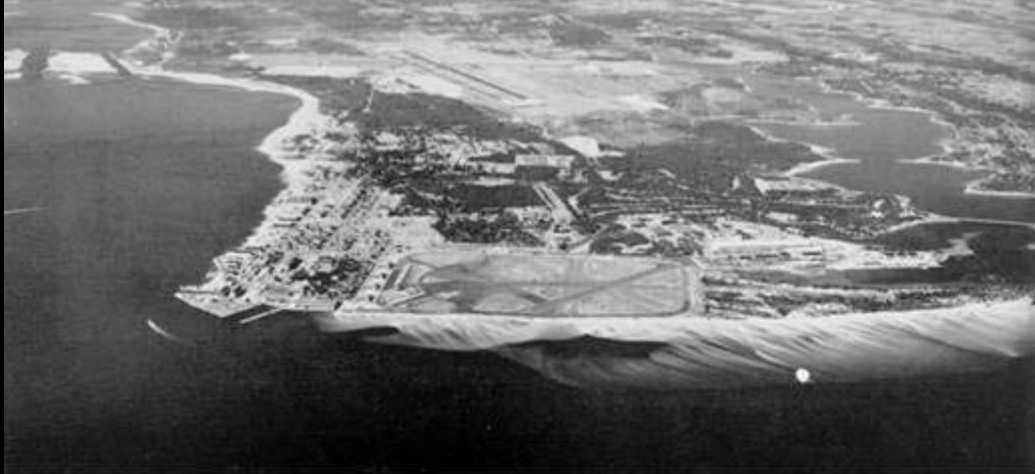
Aerial view of the Naval Air Station Pensacola shows mainbase and Chevalier Field in the foreground.
