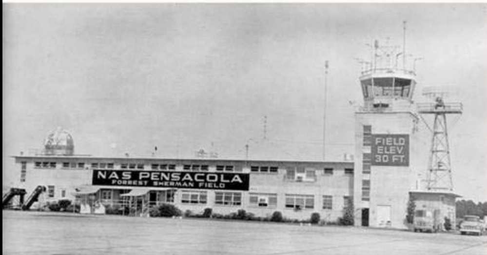
The administration building, control tower and radar scope of Forrest Sherman Field, NAS Pensacola.
