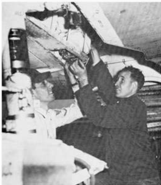
Trouble Shooters replace fuel boost pump on west line.
