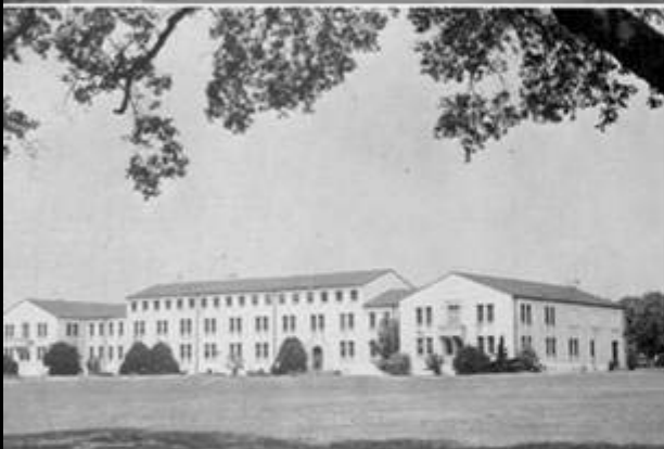
Familiar to all Navy photographers, "Building 1500" is the laboratory, administration headquarters and "home" of the Naval School of Photography.
