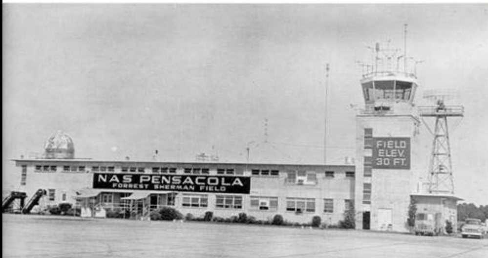
The administration building, control tower and radar scope at Forrest Sherman Field, NAS Pensacola.
