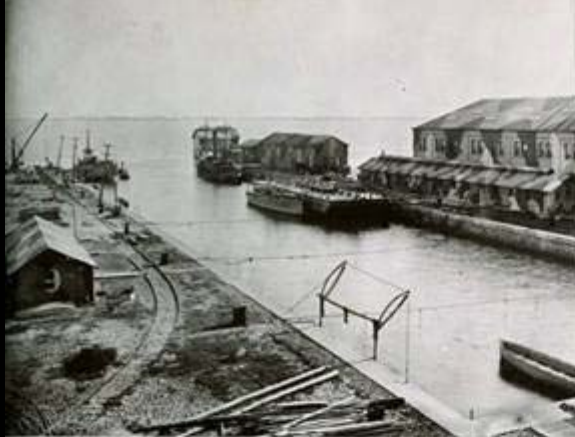
Wet Slip 1918 — and as it is today
