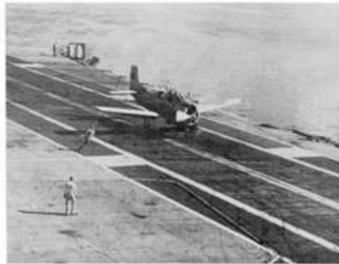
Student catching a wire on an arrested landing at the carrier.
