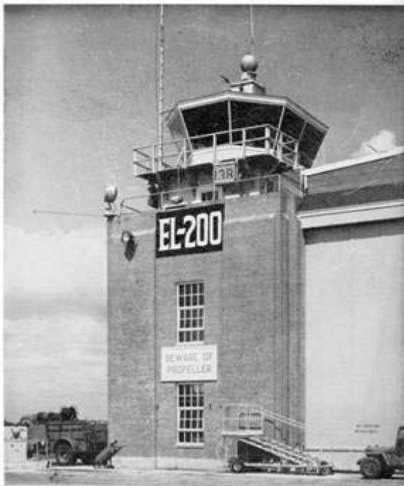
North Field Tower aboard Whiting Field.
