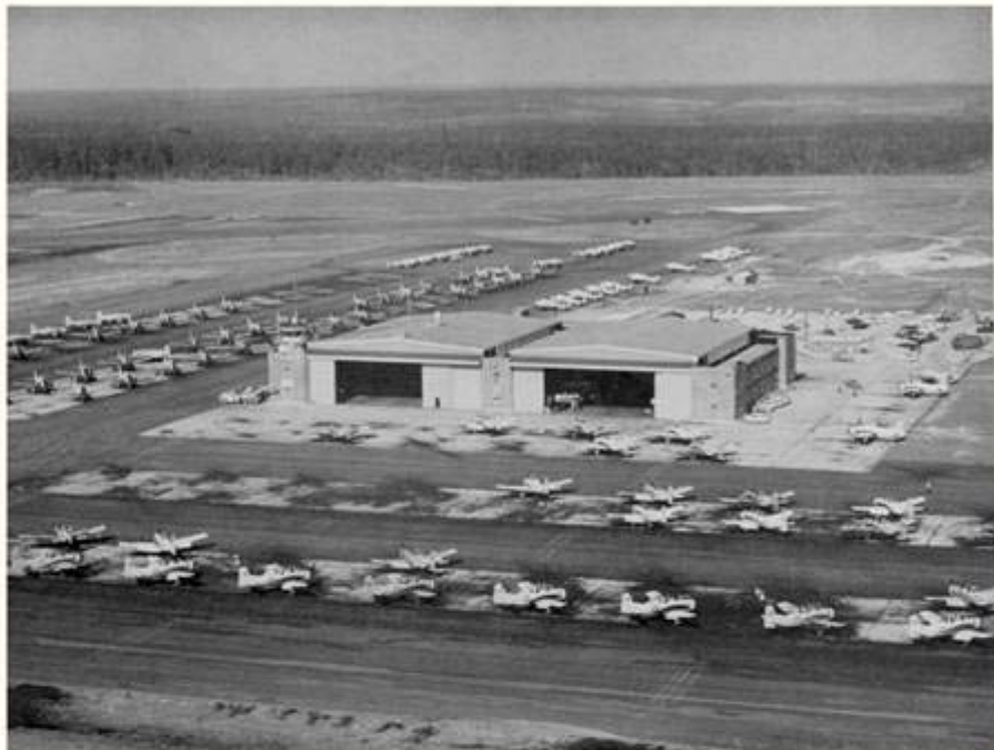
North Field hangar at NAAS, Whiting Field.
