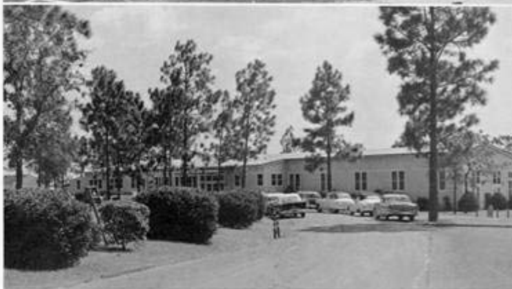
Various station buildings (O'Club)
