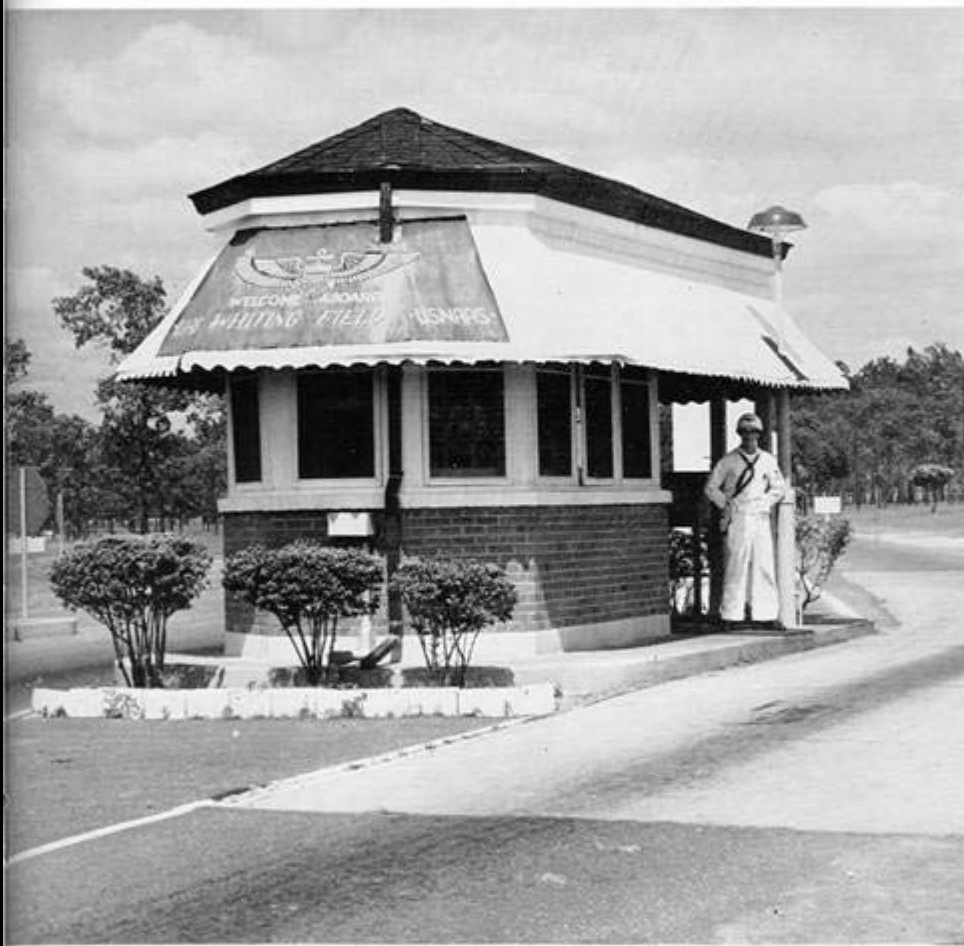
Main gate at Whiting Field.
