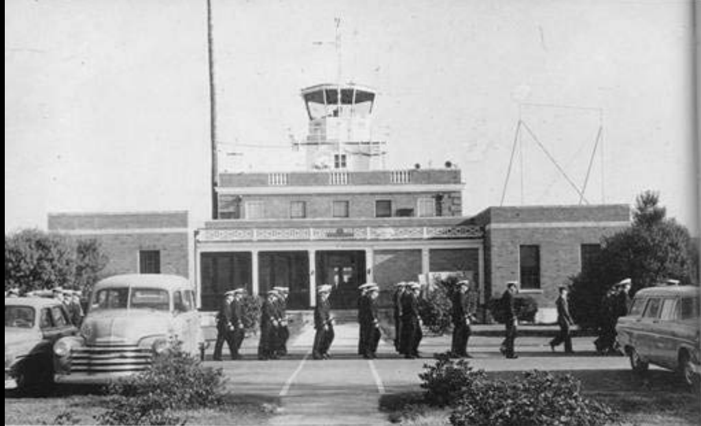
Student officers march past the administration building.
