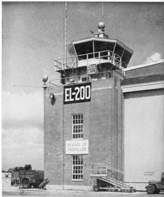
North Field Tower aboard Whiting Field.
