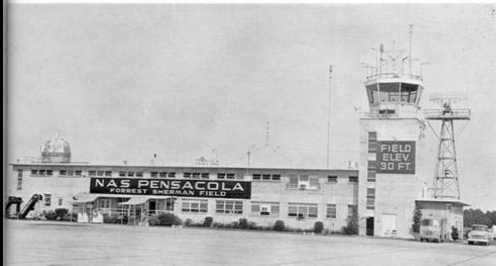
The administration building, control tower and radar scope at Forrest Sherman Field, NAS Pensacola.
