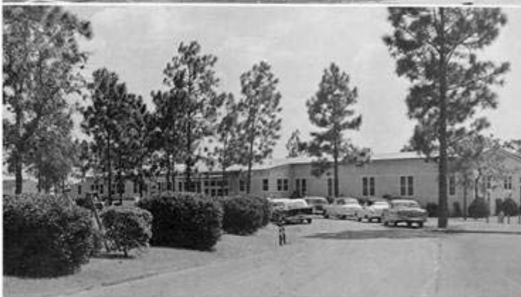
Various station buildings (O'Club)
