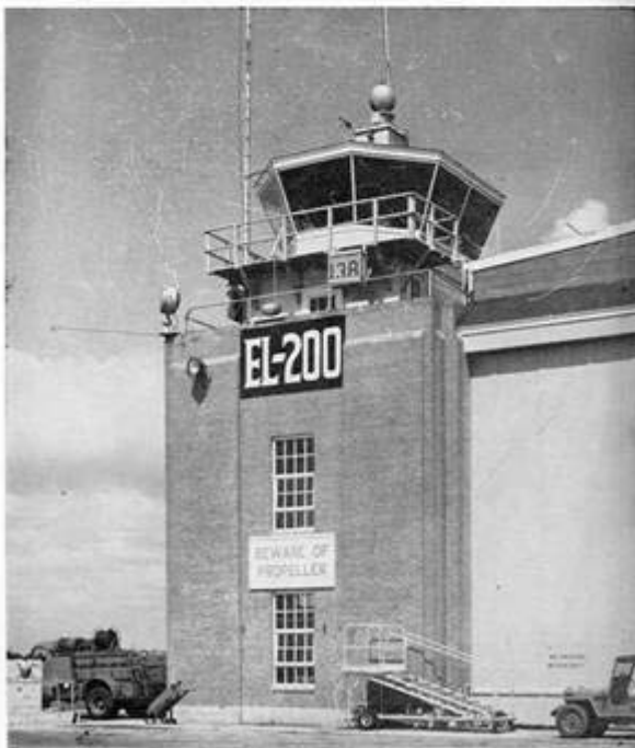
North Field Tower aboard Whiting Field.
