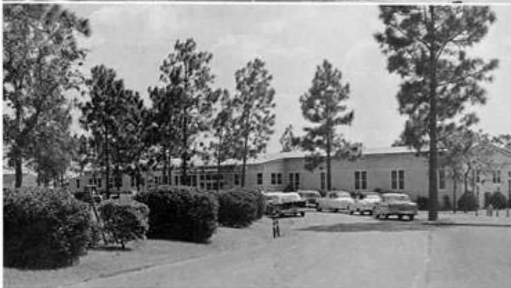
Various station buildings (O'Club)
