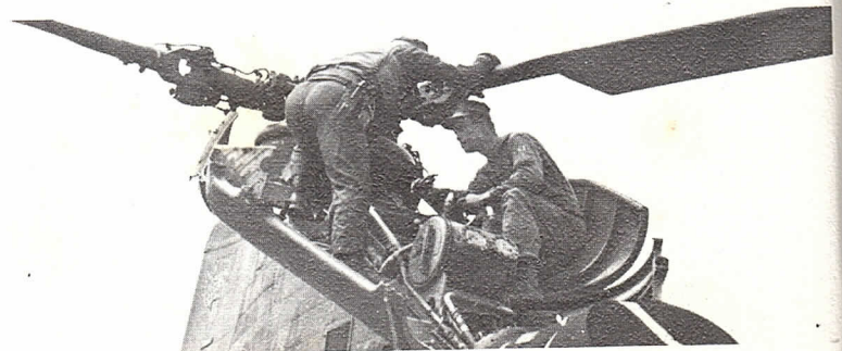
Pilot and crew chief perform the essential pre-flight inspection
