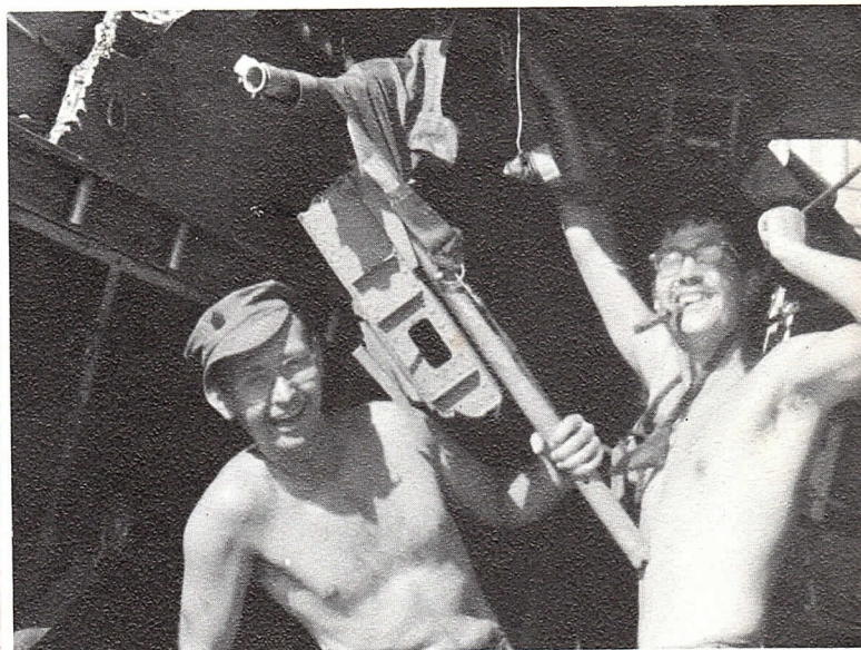
Our highly skilled and well trained Hydraulic Department on the job.
