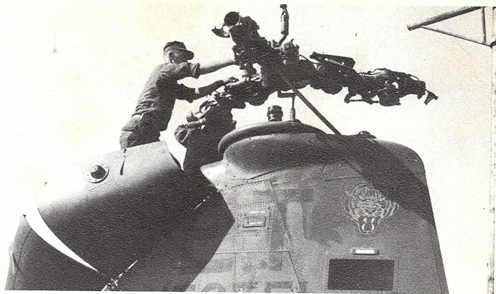
Off comes the rotor head
